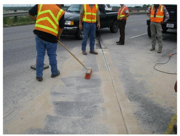
THE JOINT FILLER IS COVERED WITH SAND TO ELIMINATE TACK, THEN IT CAN BE OPENED TO TRAFFIC AS SOON AS CLEAN-UP IS DONE.
