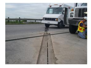
CUT & REMOVE EXISTING JOINT DOWN TO CONCRETE, AND ABOUT 8" ON EACH SIDE.
